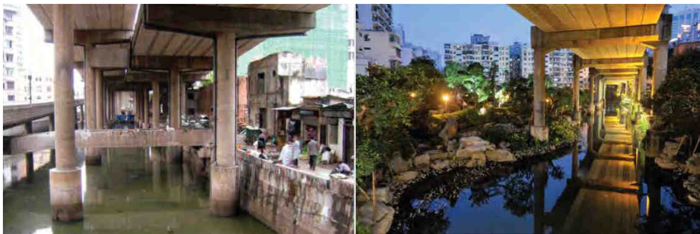
Figure 27: The Donghaochong Canal before and after restoration efforts to improve the vital public space along the BRT corridor. | Source: Far East BRT Planning Co., Limited ©Far East BRT Planning Co. Reproduced with permission from Far East BRT Planning Co.; further permission required for reuse.
