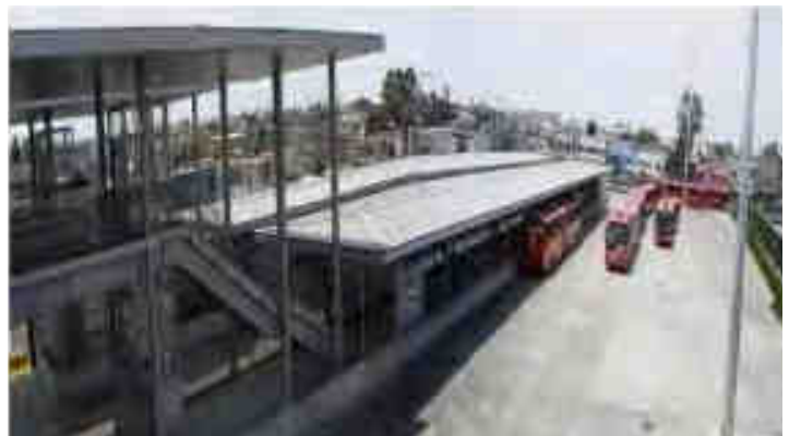
Tepalcates Central Station (After)
